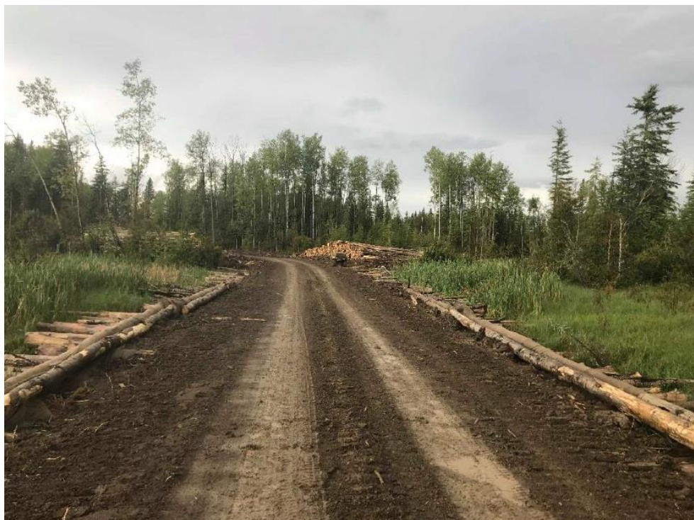
Figure 1 Typical temporary non-frozen season stream crossing.
