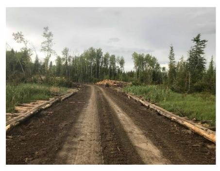
Figure 2. Temporary stream crossing in a cutblock. Modified logfill.
