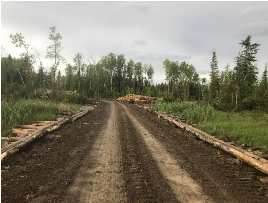
Figure 2. A typical temporary stream crossing
